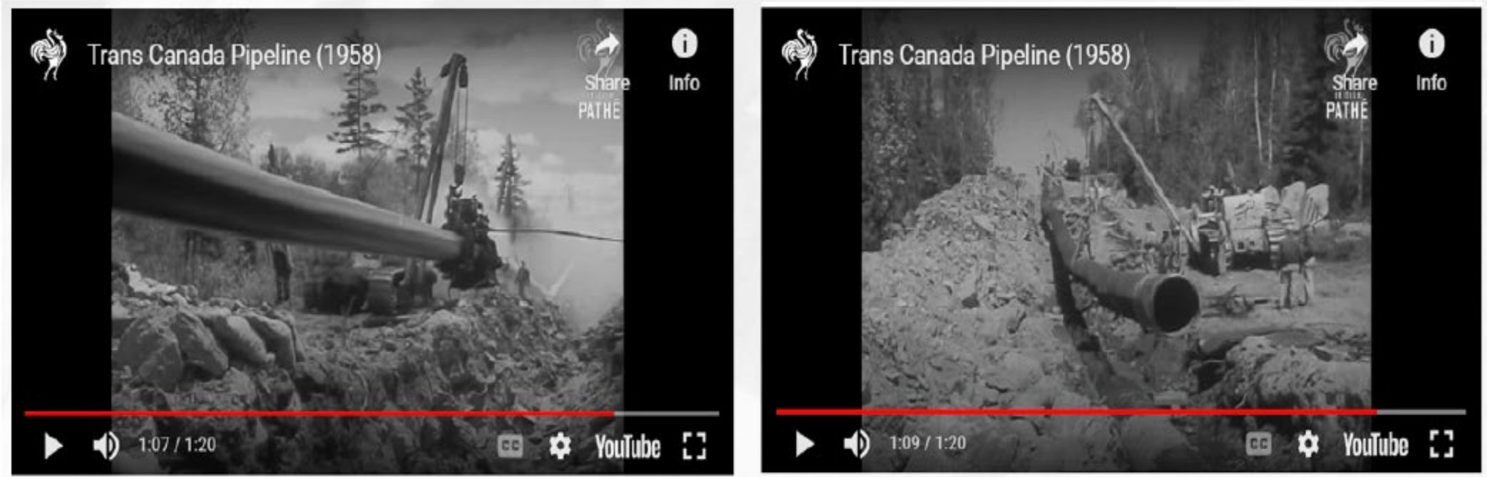
Figure 2-1 1958 Video – Canadian Mainline Canadian Shield Construction: Pipe Lowered Onto Bedrock
