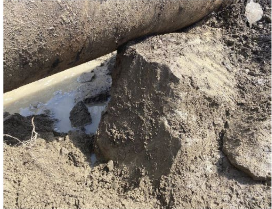
Excavation Large rock against pipe with no fractures
