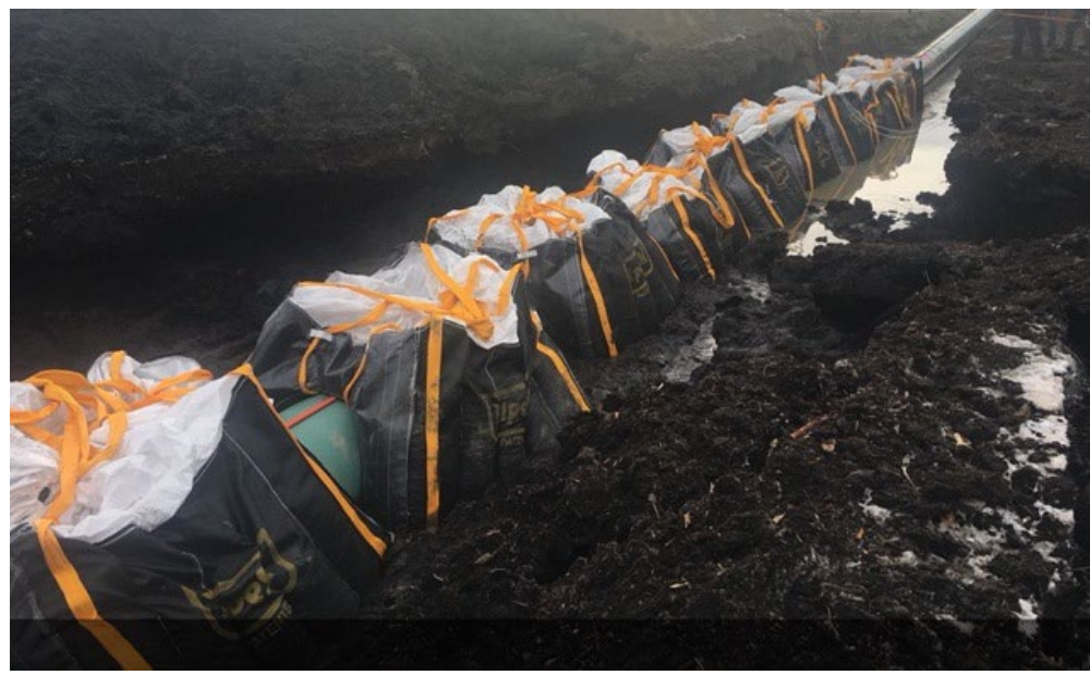
Conduit installation with weight bags
