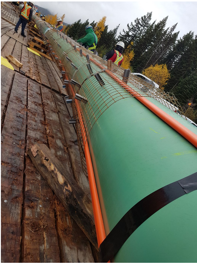
Conduit installation in concrete casing
