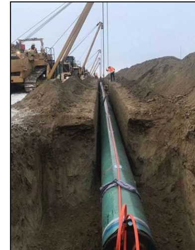
Conduit deployed On-pipe
